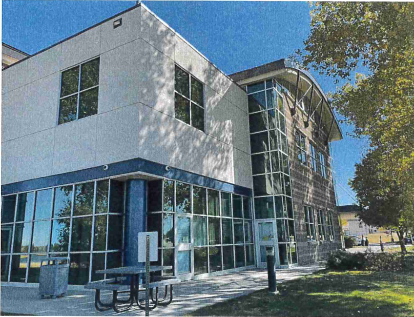
Photo 3 – View of the northwest corner of the building.
