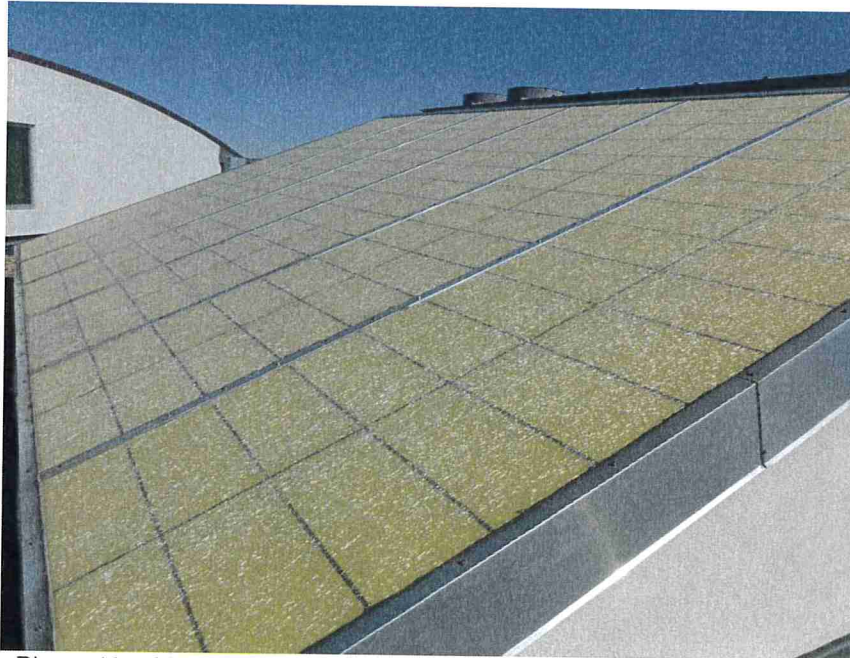
Photo 48 – View showing the skylight in the main roof area.
