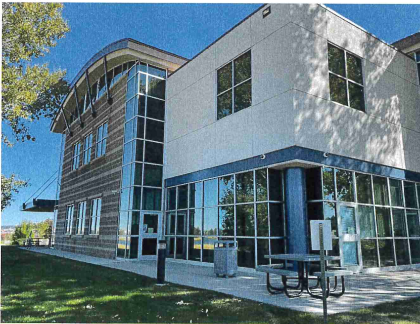
Photo 4 – View of the north elevation of the building.
