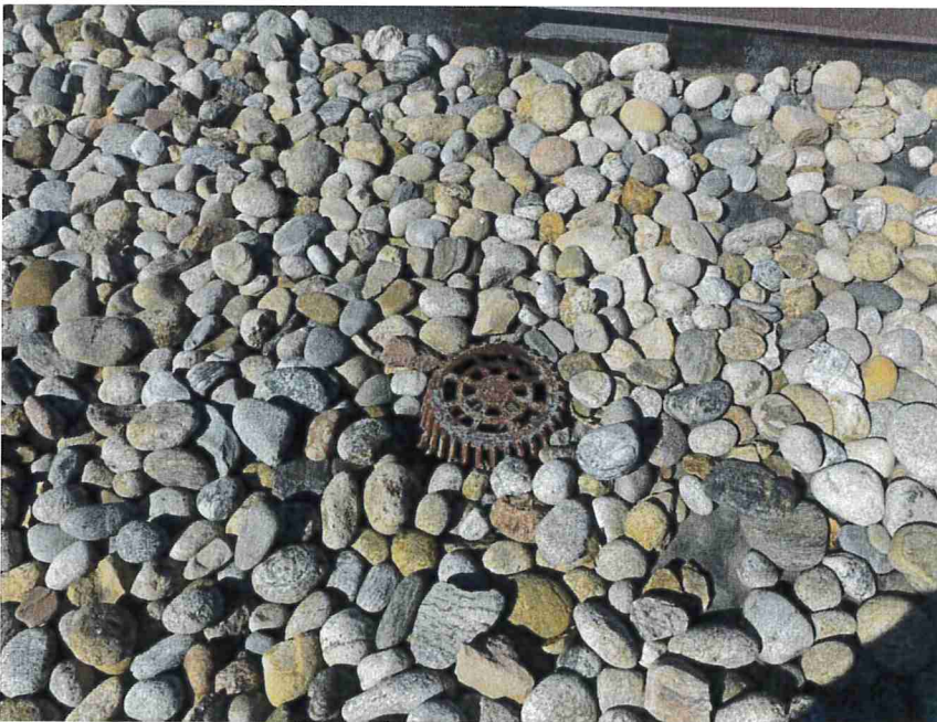
Photo 10 – Existing roof drains were clear of debris and had no signs of clogging on the roof.
