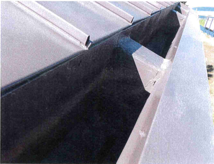
Photo 28 – Internal gutters along the standing seam metal roof had sealant joints.
