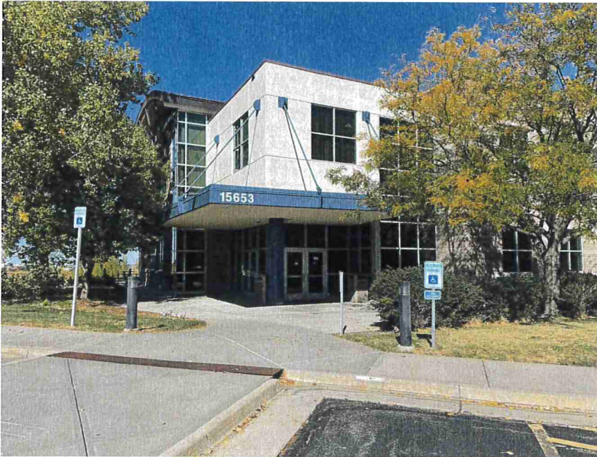
Photo 1 – View of the front (south) entrance from the south parking lot.
