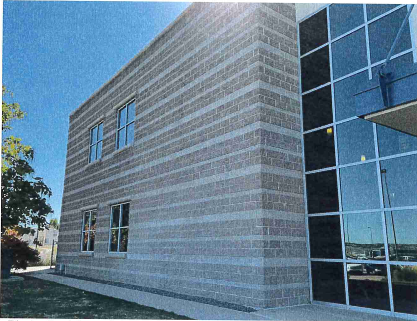
Photo 5 – View of the east elevation of the building.
