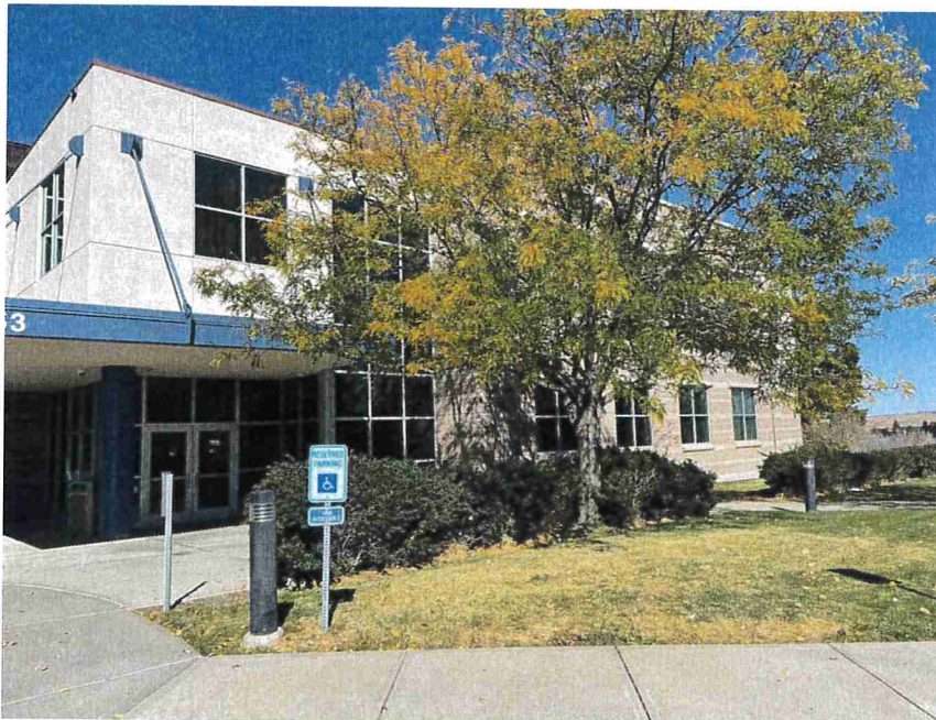
Photo 6 – View of the south elevation of the building.
