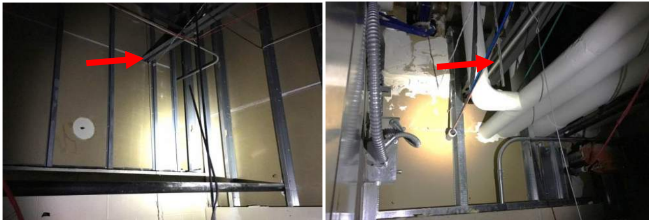
Figure 1 & 2 – Existing Non-Compliant 2-Hour Rated Wall & Construction Examples
